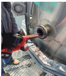
Clean flange nozzle CEMs unit 1 &amp; 2
