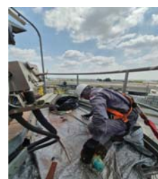
Check and clean temperature sensor unit 1
