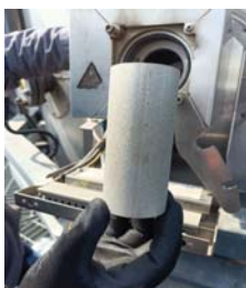
Clean filter probe CEMs unit 1 &amp; 2
