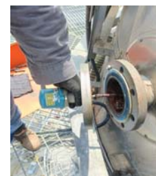
Check and clean temperature sensor unit 2
